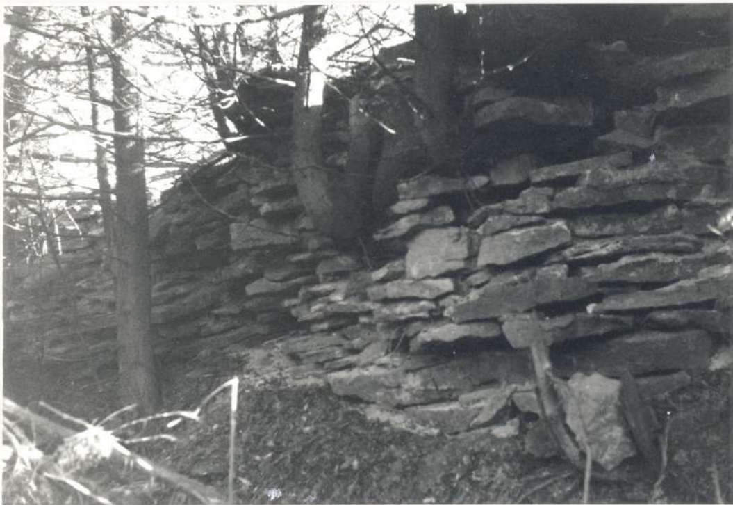
29. upper: site of lock four lower: rubble masonry walls at lock four — either support of wooden lock or masonry replacement (photos by author)
